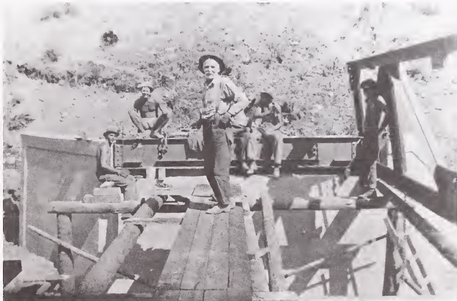
Civilian Conservation Corps crew constructing the Fishtail Bridge in northwestern Montana, 1934. (Vurl Springer).
